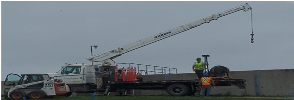
Staff utilizing the boom truck to remove a SBR Recirculation Pump
