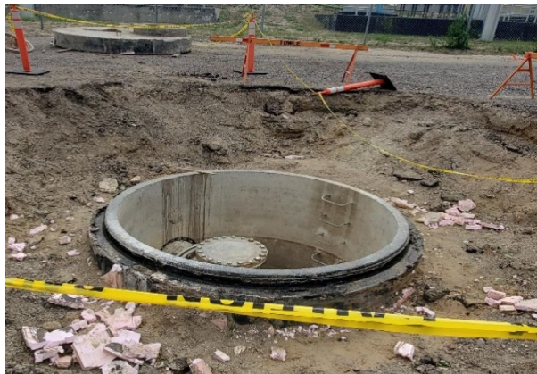
Clean out of Poplar Bluff connection point
