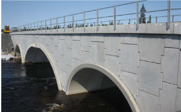
Figure 7: Sample Open Bottom Arch Culvert
