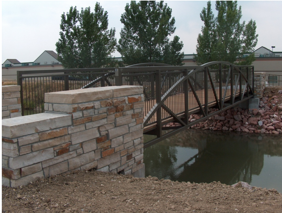
Figure 10: Sample Steel Truss Active Transportation Bridge
