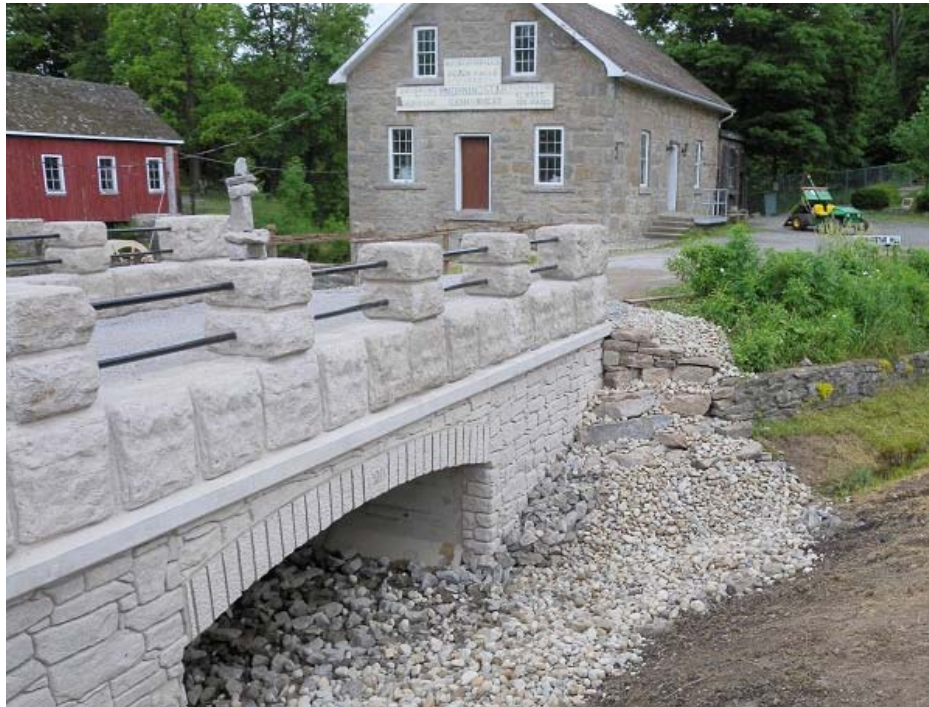
Figure 9: Sample Box Culvert
