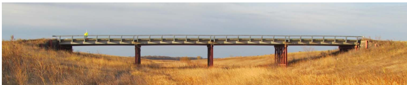
Figure 6: Sample Prestressed Precast Concrete Girder Bridge
