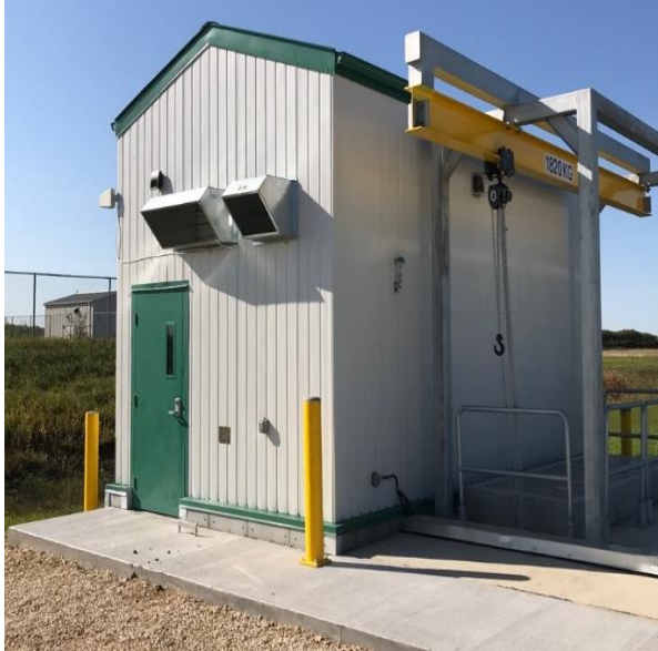
Poplar Bluff Lift Station- Exterior
