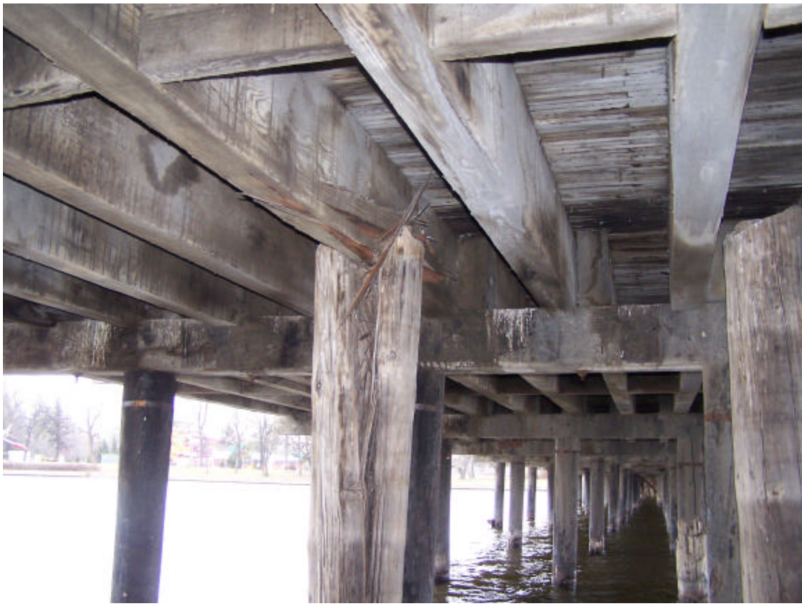
Photo 23 – Pile (jacking up)
