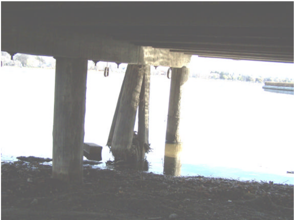
Photo 1 – Pile (broken)
