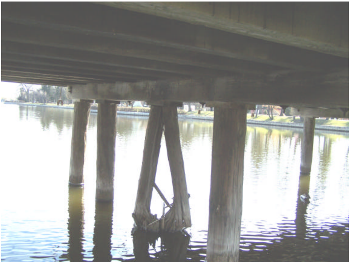
Photo 9 – Pile (broken)
