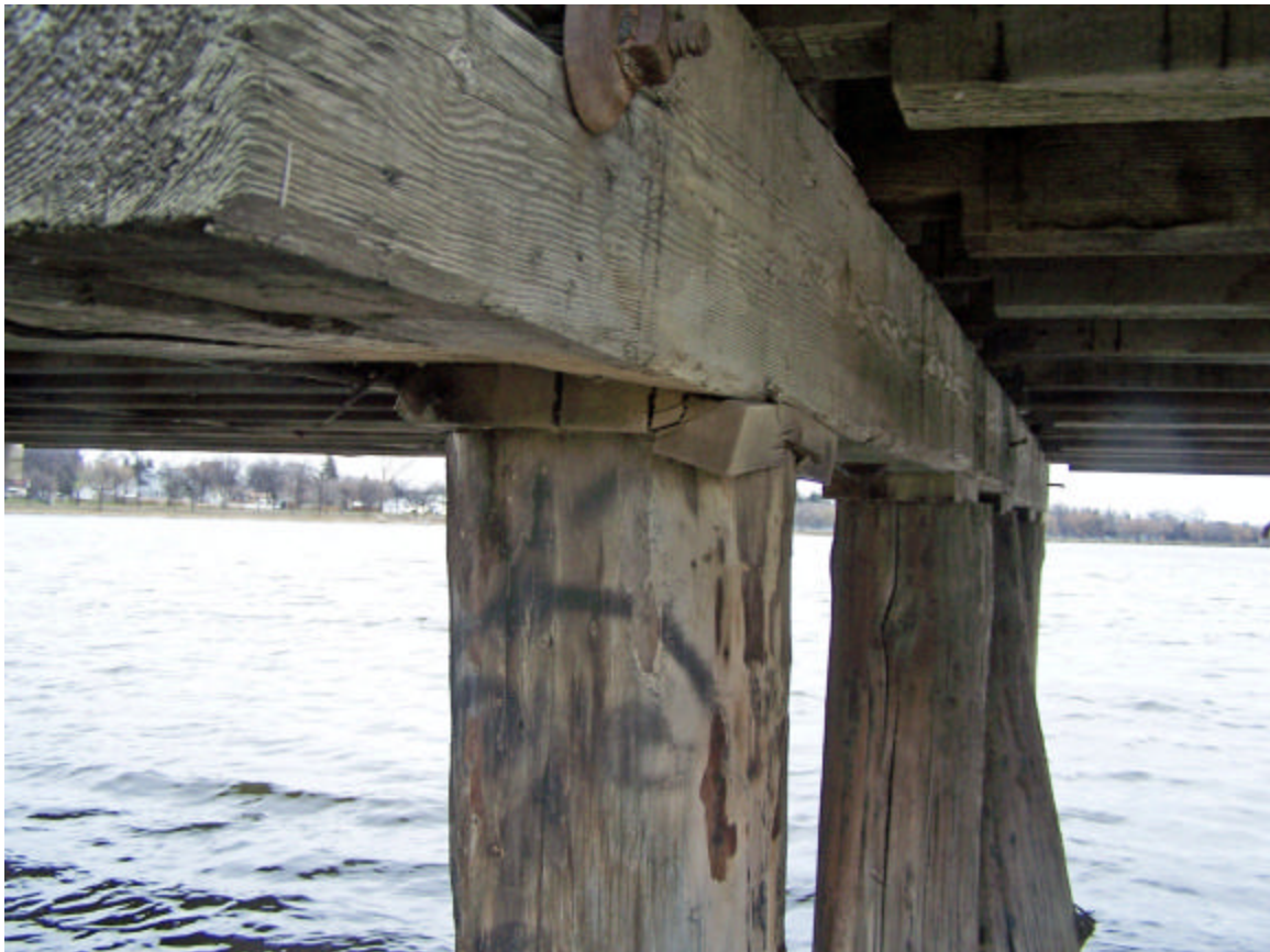
Photo 8 – Pile (jacking up, crushing shim)
