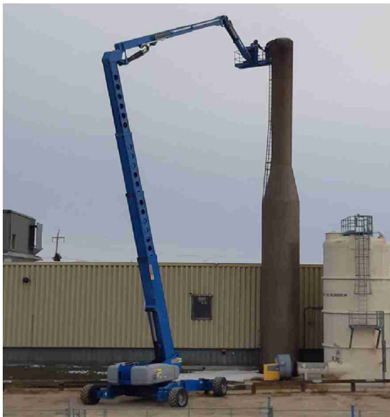
Light beacon replacement using lift
