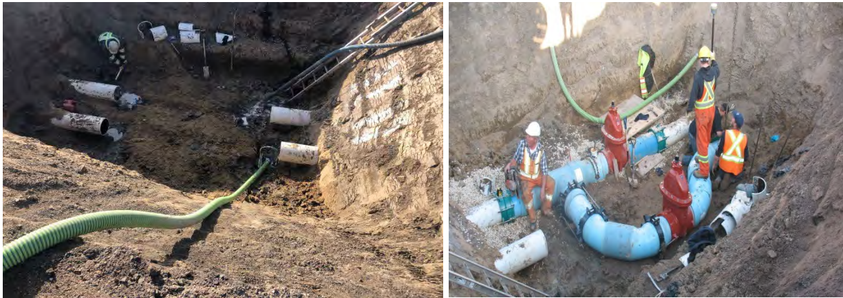
Poplar Bluff North and South Force mains – before and after connection
